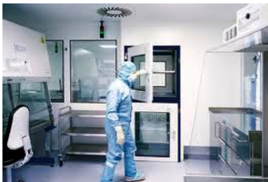
Fig. 28.4. Laminar air flow room
